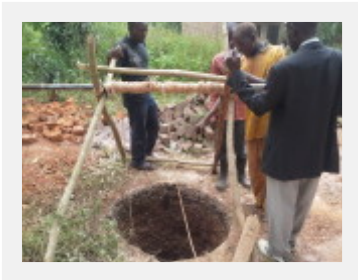
Is well hand digging at the new school.
