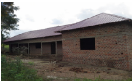
New School Building Kampala
