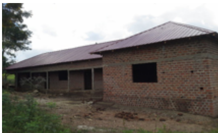
New School Building Kampala
